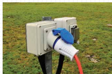
Every pitch at Holgates Caravan Park at Silverdale has a 16-amp power supply; you still have to calculate the amps you use, though.
